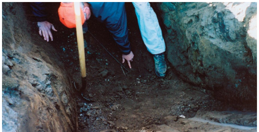
Troy Hayes points to the top of Mile 50 West. The original monument was recovered six feet below the surface of the existing road.
