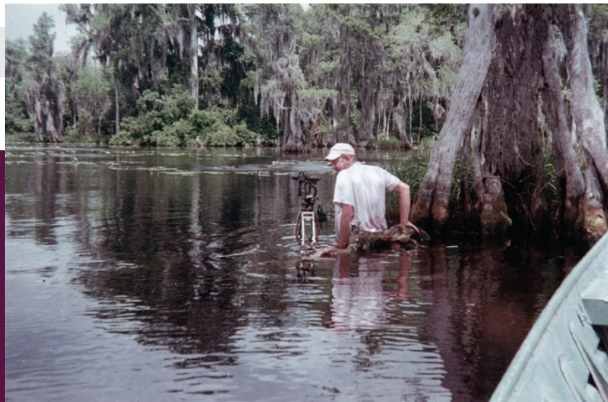
Surveyor Gus Hart (Bill's brother) wades through a swamp with his equipment during the initial surveying for Walt Disney World. Photo courtesy Bill Hart, Jr.
