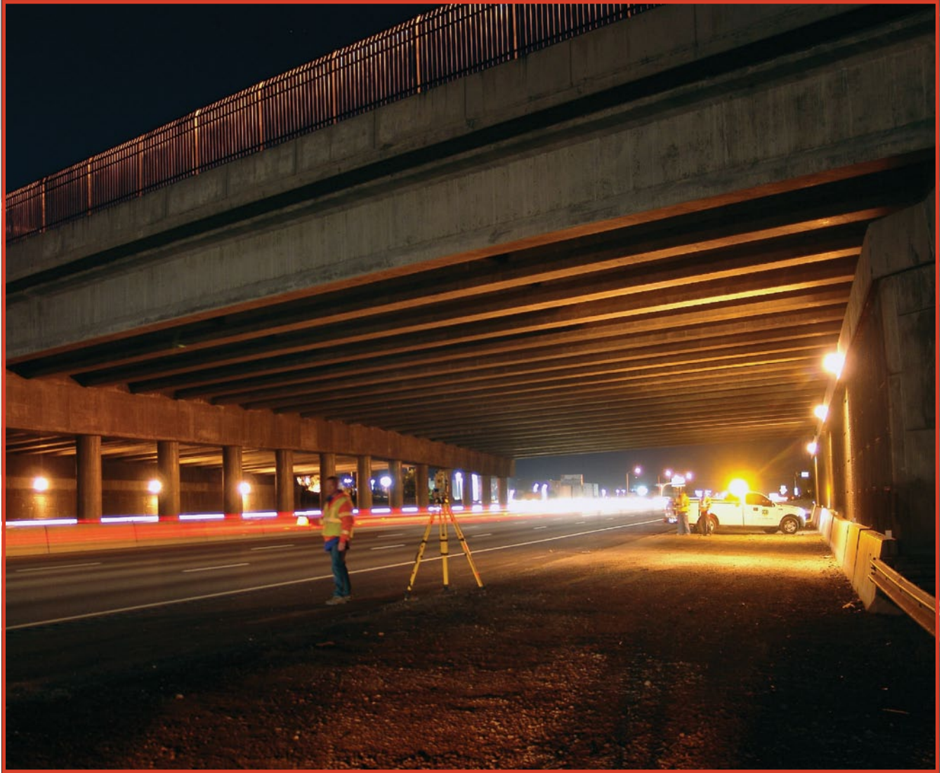
Much of the surveying was done at night, under traffic, which required extra workers to protect the crews.
